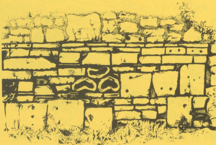
Wall in Crews Hole Road
